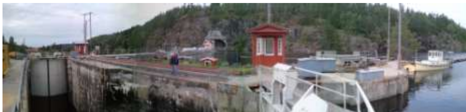
Svanedam locks and Tistedalsfoss hydropower station
