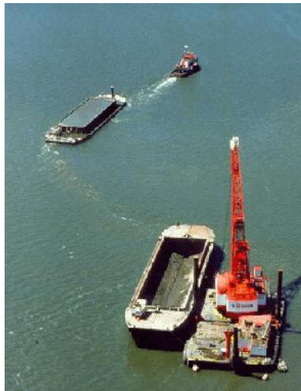
Removal and transport of contaminated bottom sediment
